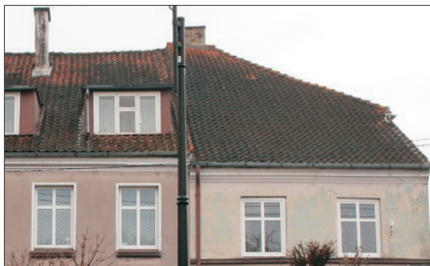
Fig. 9. A mansard roof
