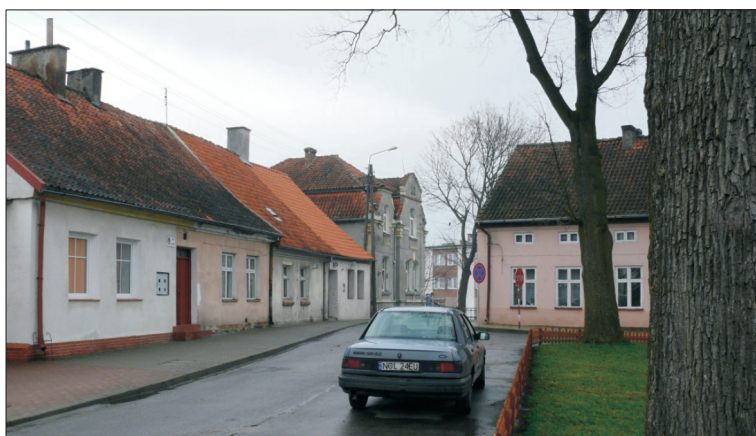
Fig. 9. Castle Square – the north frontage
