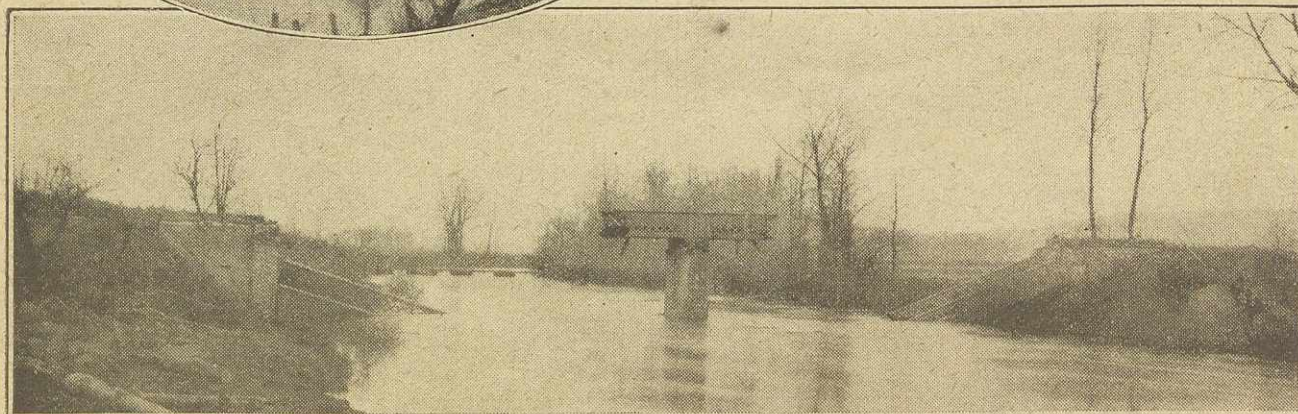
The central pier of another bridge over the Aisne, with a fragment of the ironwork still in position. The pity of all this destruction seems to be the utter needlessness of it. While justifiable according to military law, it failed to cause the delay which was its purpose.
