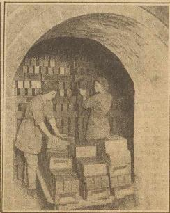
Work at the world's largest brick kiln, near Peterborough. To the left women are unstacking bricks and putting them on the slide down which they travel to a railway waggon. On the right they are stacking bricks in a kiln ready for firing.
