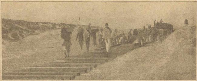
Laying a railway over the desert. As the British advanced the engineers spun lines behind them, light railways and broad-gauge tracks linking the base with the vanguard, ever progressing towards Palestine, and bringing up materials for still further lines.
