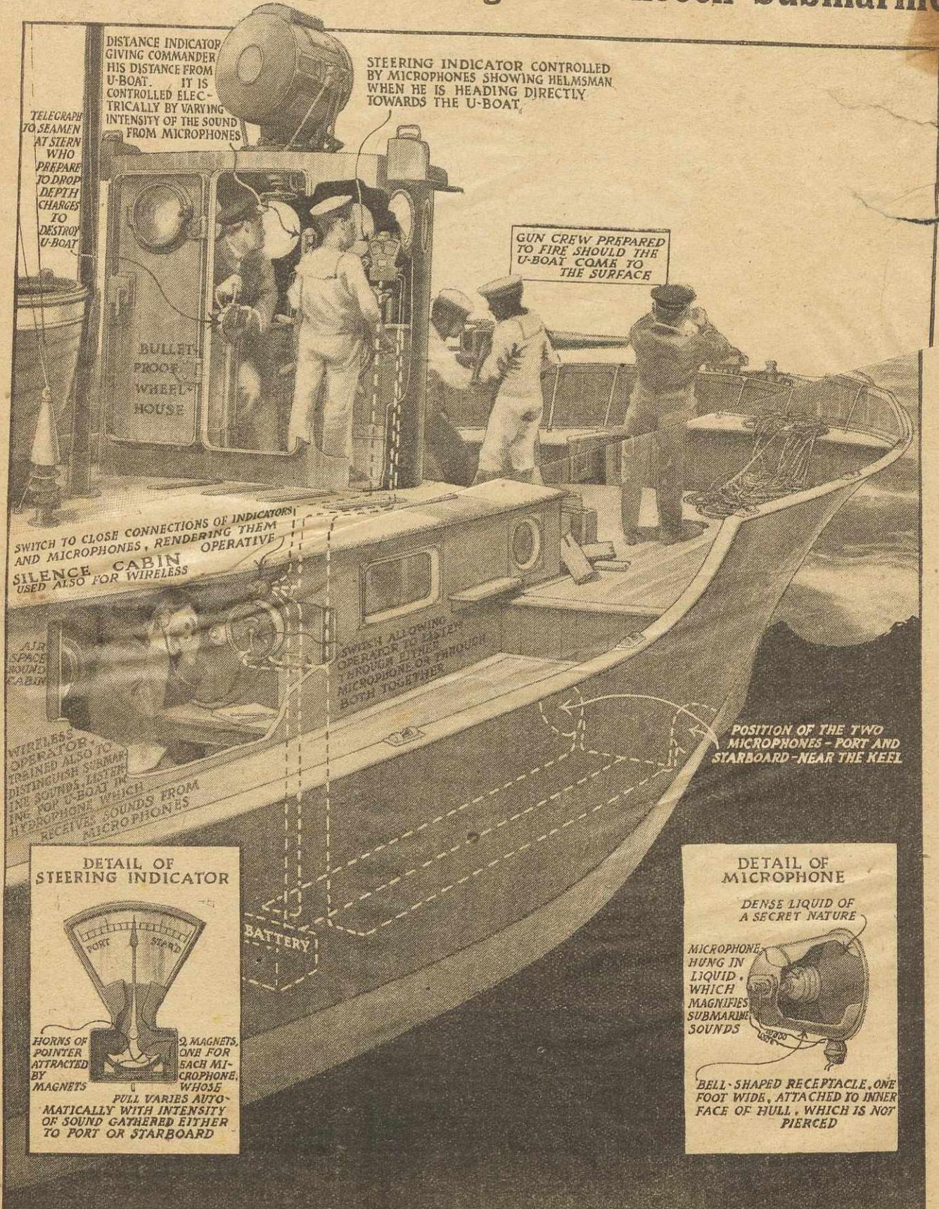
DISTANCE INDICATOR GIVING COMMANDER HIS DISTANCE FROM U-BOAT. IT IS CONTROLLED ELECTRICALLY BY VARYING INTENSITY OF THE SOUND FROM MICROPHONES
